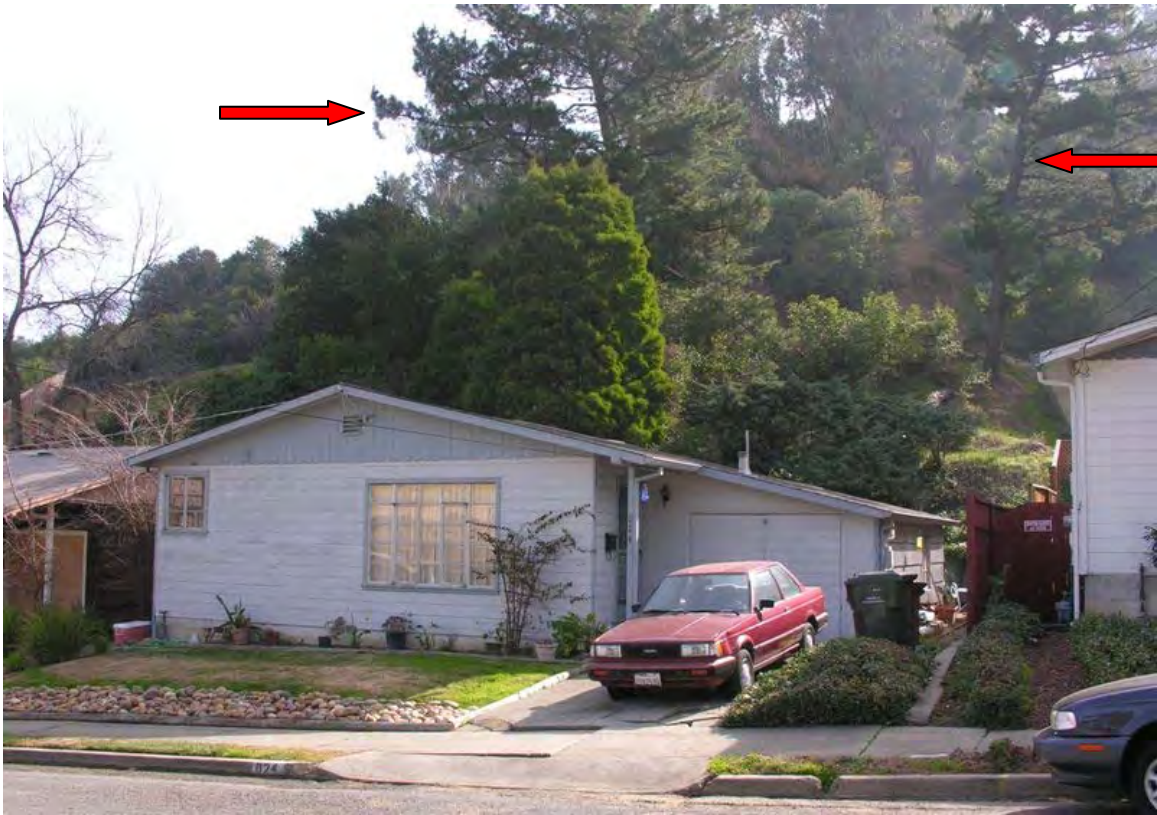
Front Detail. Arrows point to pines tagged for removal.
